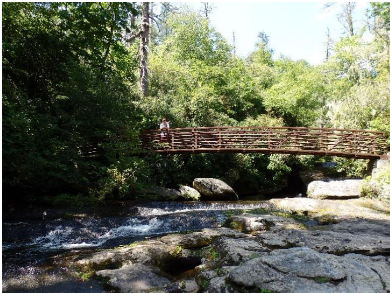
Steel Bridge over a Chattooga Tributary
