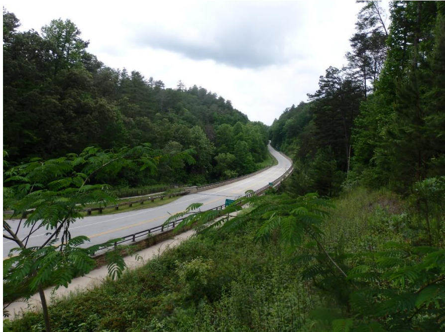
The Highway 76 Bridge
