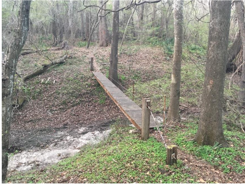
Bridge Over Mitchell Creek
