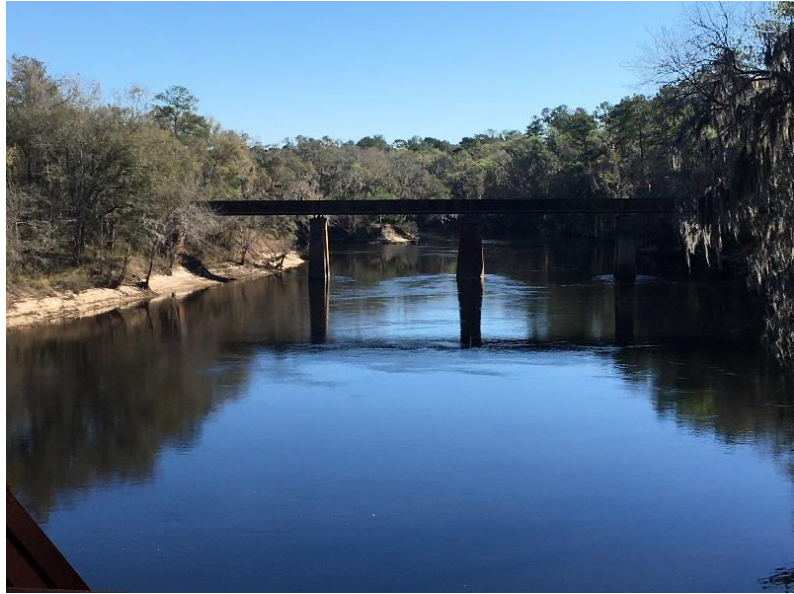
Looking Upriver from the Abandoned U.S. 90 Bridge
