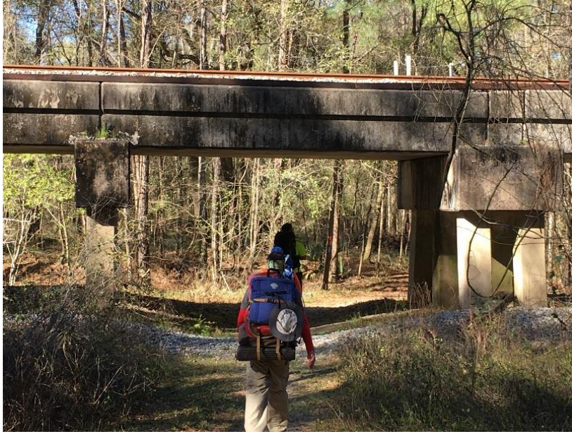
Crossing under the Railroad
