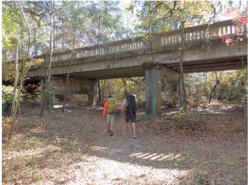
Crossing Under the Old U.S. Highway 129 Bridge
