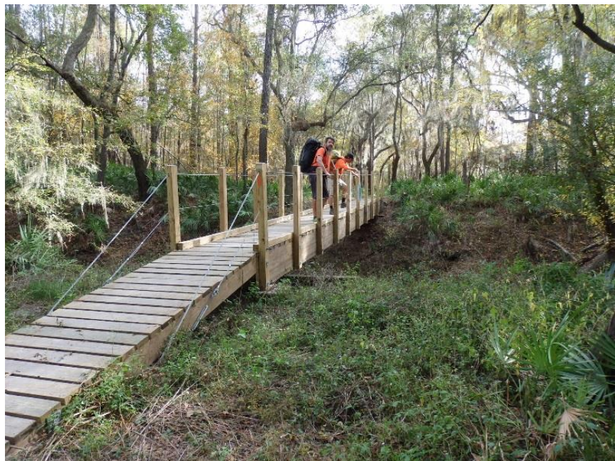
The Elaborate Bridge over Swift Creek
